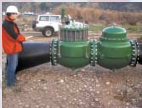
Assembly at site of Fig. 2010 DN500 Globe type Strainer, upstream of a pressure reducing control valve.
